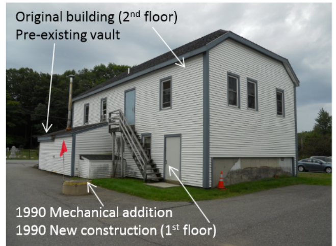
2) Exterior – East (left) and north (right) facades; original 1-story school house building was lifted and added on to in 1990
