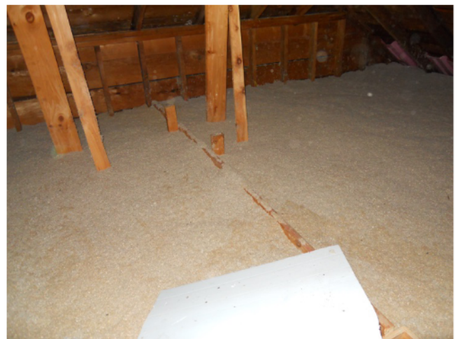
6) Ceiling framing – Ceiling joists require intermediate support; haphazard verticals provide additional support in some locations
