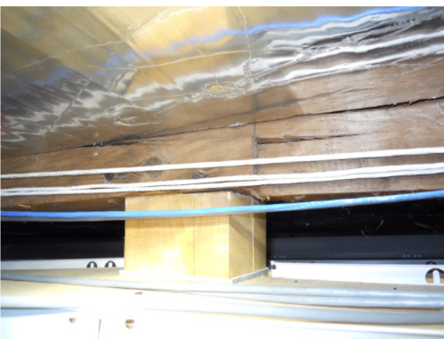
11) Second floor framing – Existing dropped 6x6 beams are severely deficient; cracked beam near southeast post is structurally compromised
