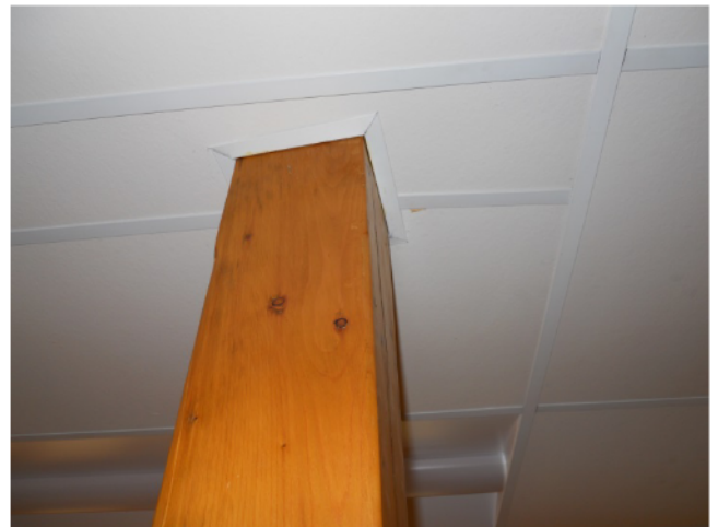
16) Second floor supports – Northwest post in meeting room is severely bowed, skewed and moderately checked; replacement required
