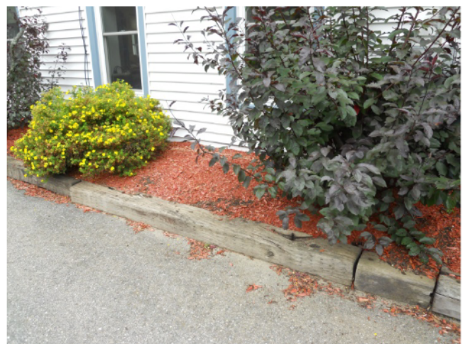
36) Exterior – Raised beds against the structure increase the presence of moisture; lower beds and regrade to slope away from the building
