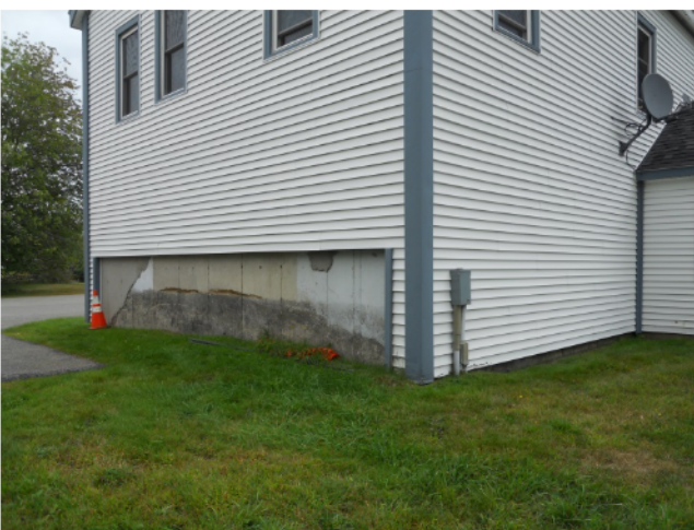
23) Foundation – North foundation; grades have been lowered on exterior; wall is bowed inward and has been previously repaired
