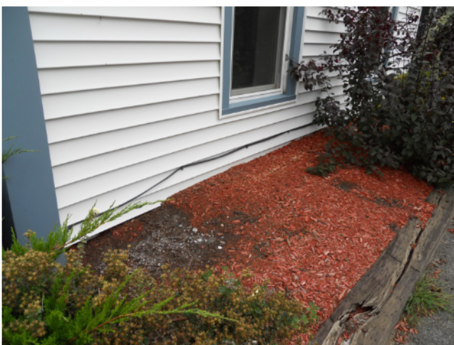
35) Exterior – Raised beds against the structure increase the presence of moisture; lower beds and regrade to slope away from the building
