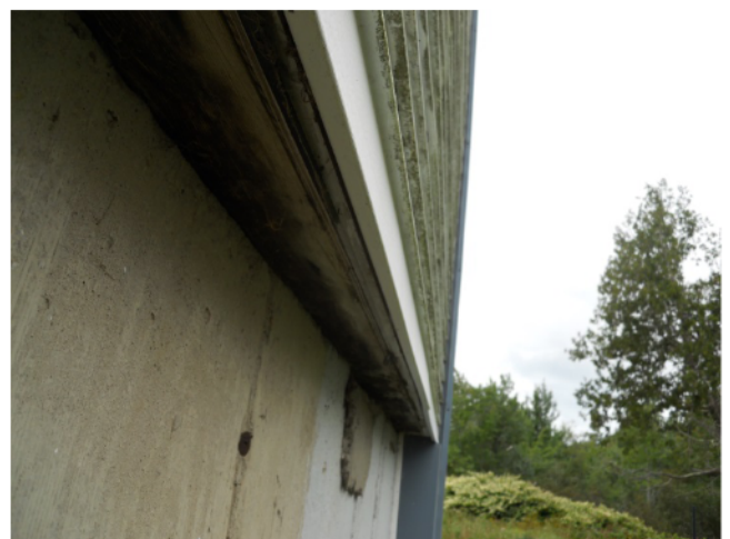
24) Foundation – North foundation; wall is significantly bowed inward
