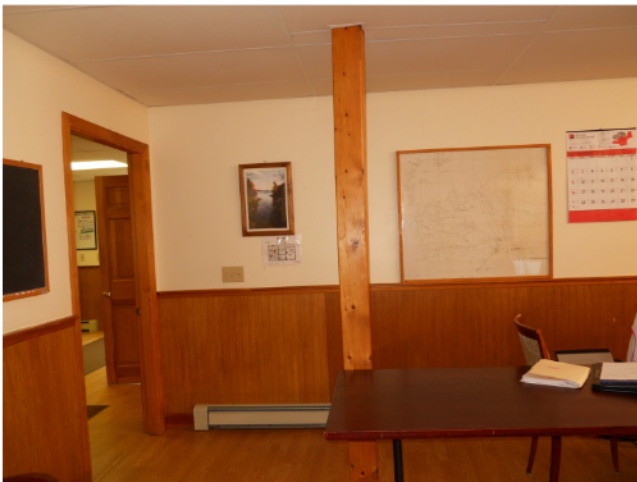
15) Second floor supports – Northwest post in meeting room is severely bowed, skewed and moderately checked; replacement required
