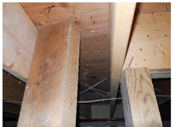
18) Second floor supports – Some posts in the crawl space may not be properly aligned with posts supporting the second floor above
