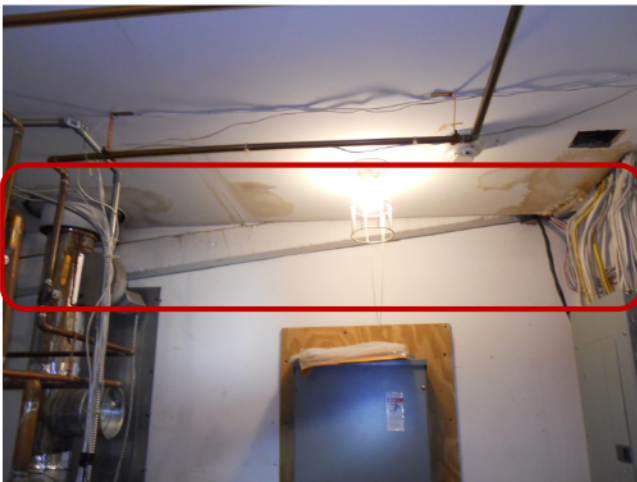
27) Vault roof/ceiling – Edge of vault roof is exposed concrete; mechanical room roof framing is not exposed
