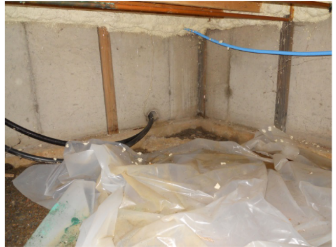
26) Mechanical room – Moisture from dirt floor should be mitigated
