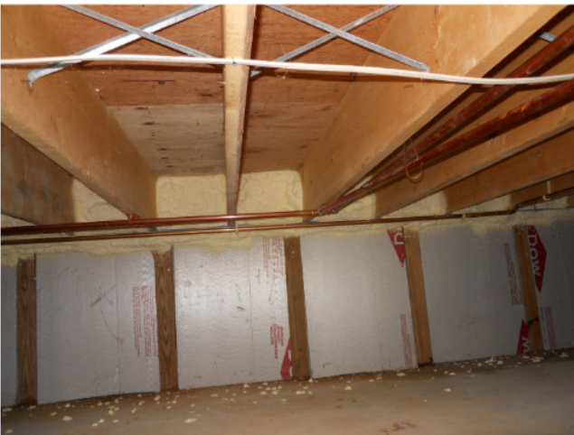
21) First floor framing – Framing at foundation wall is attached to ledger which is supported by flatwise 2x4s; rigid insulation obscures foundation
