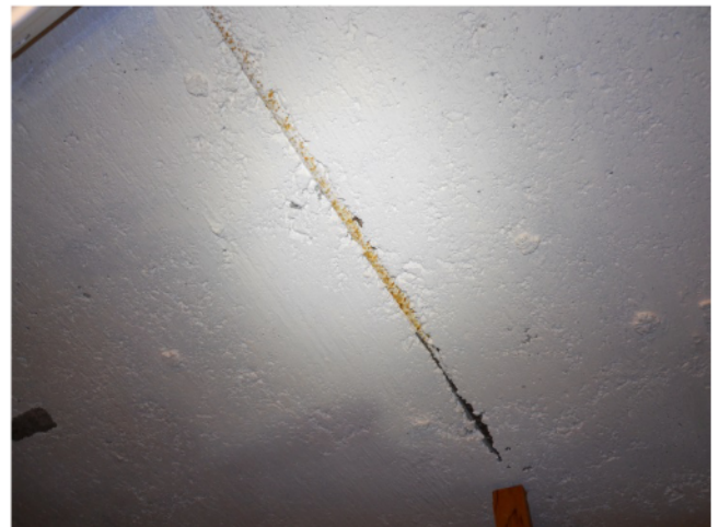
28) Vault roof/ceiling – Poorly consolidated concrete is present; rebar is exposed on underside (inadequate concrete cover)
