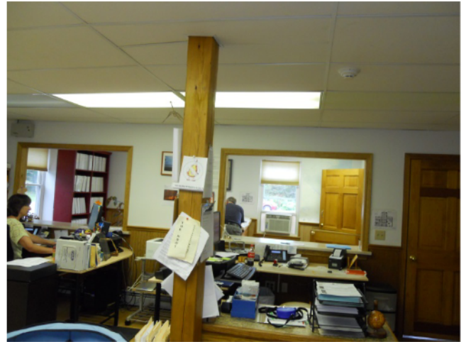
14) Second floor supports – Southeast post (foreground); beams and posts supporting second floor are recommended for replacement
