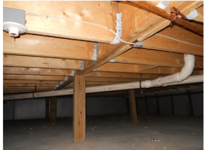
20) First floor framing – (3) 2x12 center support beam; beams is lapped and spliced; 4x6 PT support posts are spaced approximately 8' o.c.
