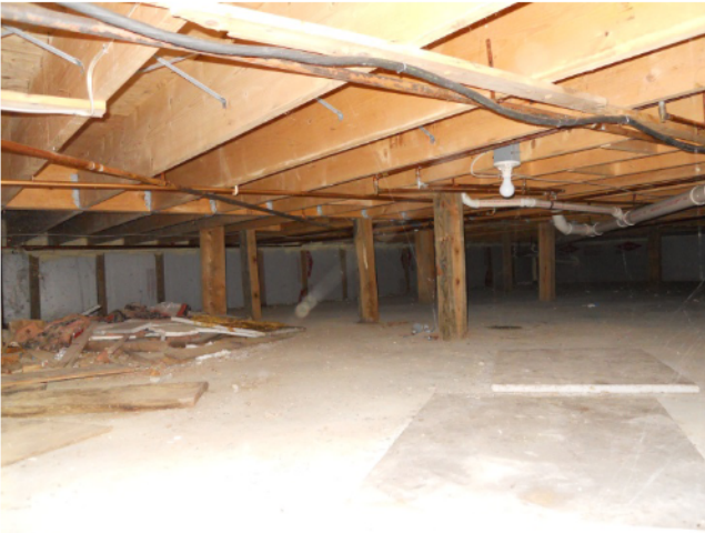
19) First floor framing – Typical framing is 2x12s at 16" o.c. spanning from exterior foundation wall to center support beam
