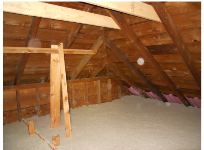
4) Roof framing – Raised south endwall with hip rafters at corner; rafter vents are present along east and west eaves due to thick insulation
