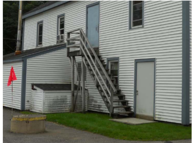
32) Exterior – Egress stairs and landing are structurally deficient; replacement recommended
