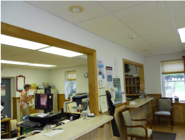
13) Second floor supports – Original post location is at window; interior wall is likely acting as an inadvertent bearing wall
