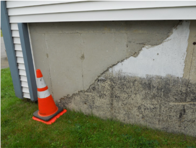
31) Exterior – Foundation repairs are evident; panel forms indicate more recent construction than 1932
