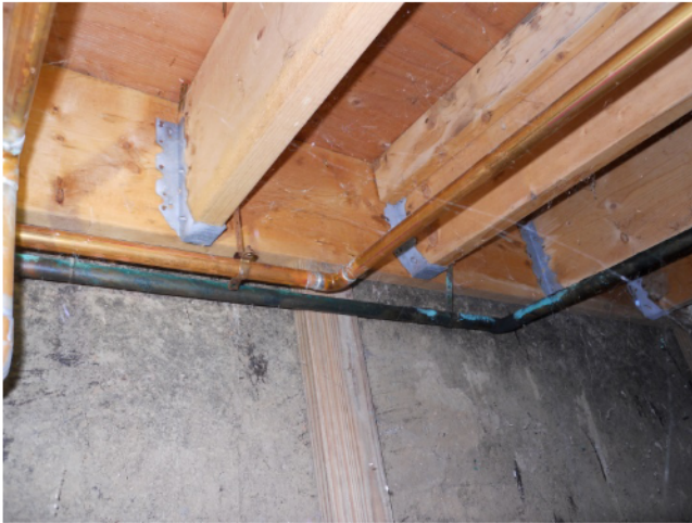
25) Mechanical room – Framing at mechanical room is sturdy, but ledger attachment is marginal
