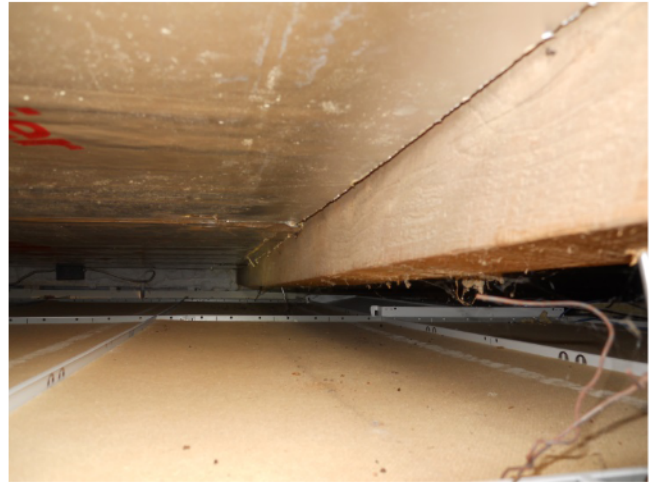
8) Second floor framing – Existing dropped 6x6 beams are severely deficient (beams are partially hidden by rigid insulation and strapping)
