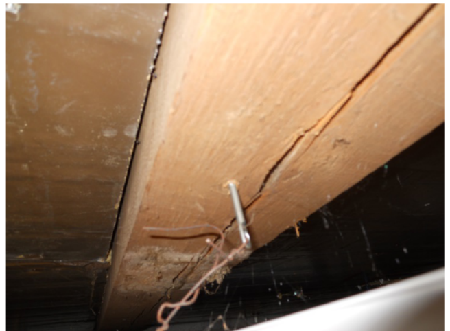
10) Second floor framing – Existing dropped 6x6 beams are severely deficient; beam cracks are likely structural
