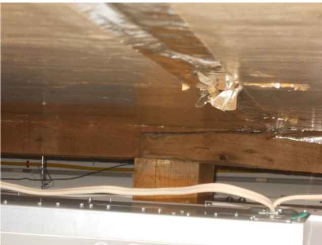
9) Second floor framing – Existing dropped 6x6 beams are severely deficient; beams are spliced at post locations
