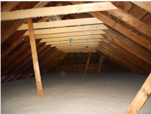
3) Roof framing – Original rafters (darker) remain; 2x6 collar ties were added to stiffen and reinforce original roof assembly
