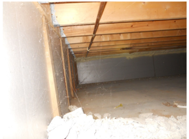
22) First floor framing – Framing at foundation wall is attached to ledger which is supported by flatwise 2x4s; rigid insulation obscures foundation
