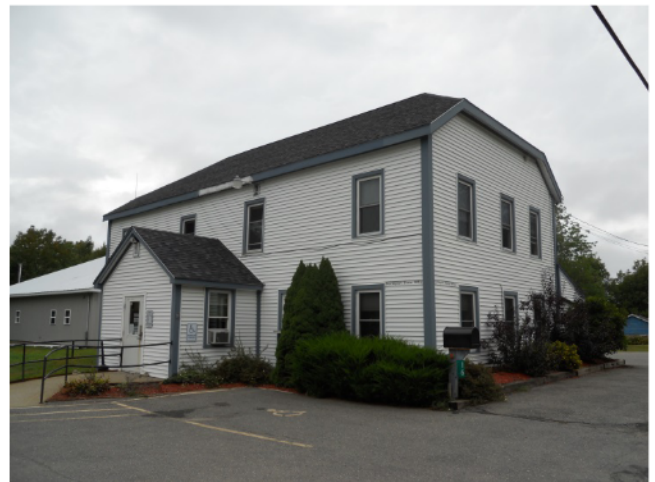
34) Exterior – Plantings adjacent to structure increase presence of moisture
